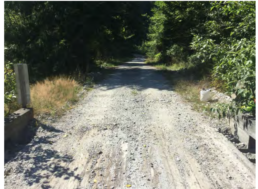
Right Approach Facing Away From Bridge
