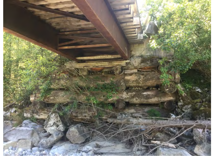
Right Bank Abutment
