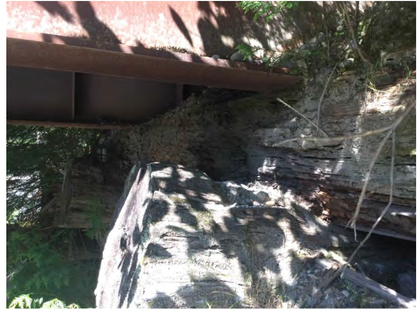
Left Abutment Top Crib Log
