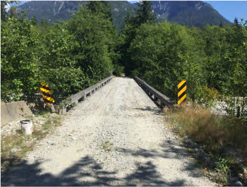
Left Approach Facing Bridge
