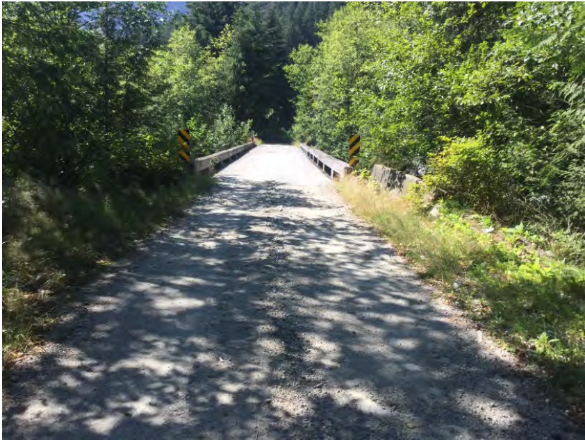
Left Approach Facing Bridge
