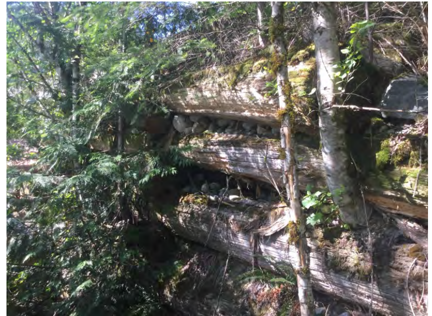
Left Abutment Downstream Wing Wall
