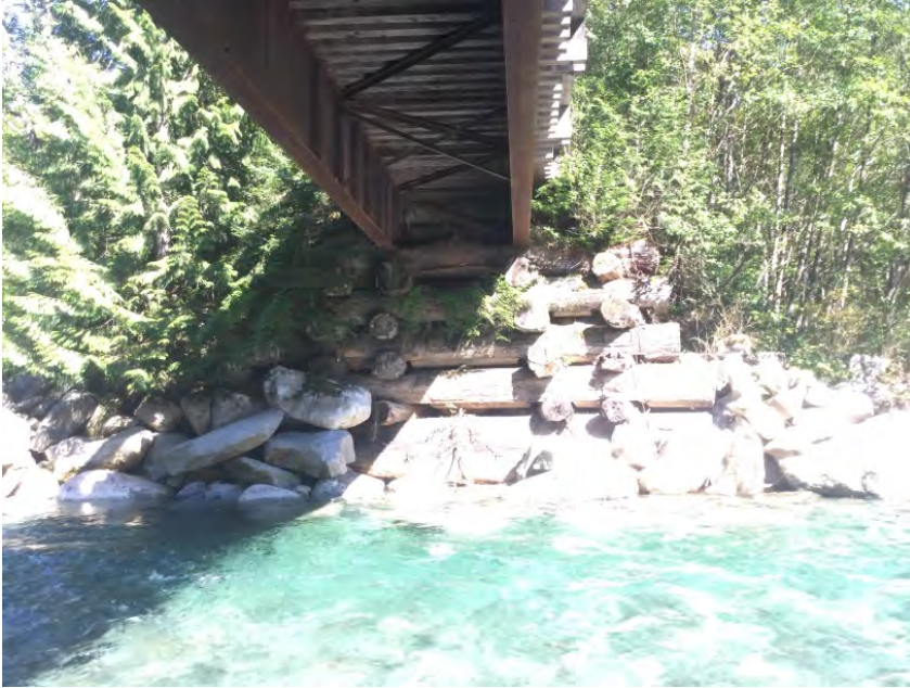
Left Bank Abutment
