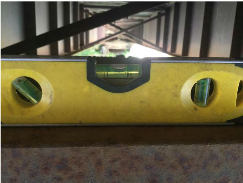
Steel Plate between Pier Posts Level
