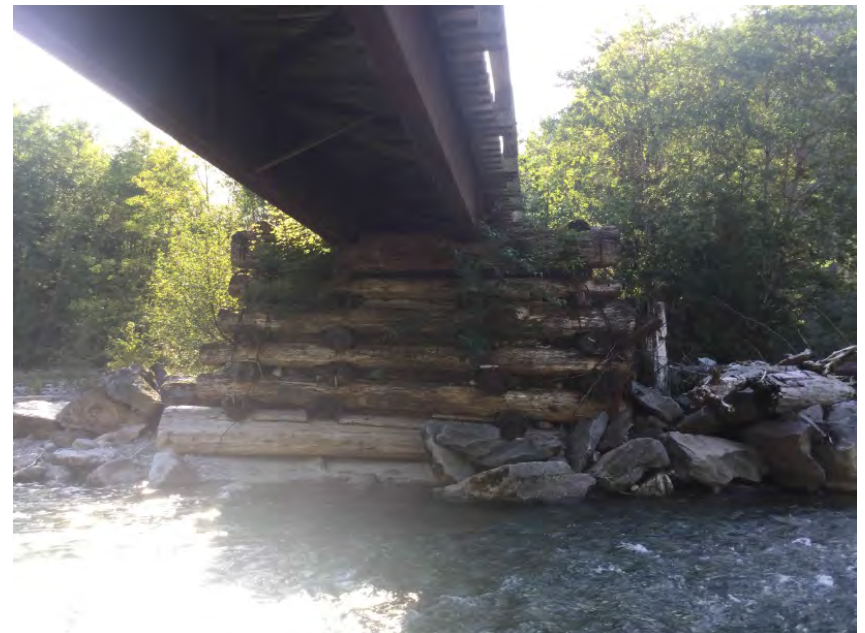
Pier Left Face
