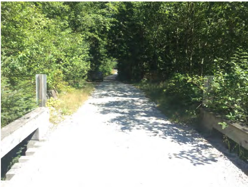
Left Approach Facing Away From Bridge
