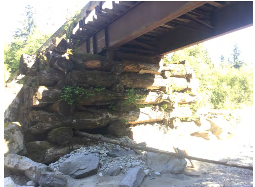
Pier Right Face
